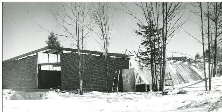
Above: Yarmouth High School under construction, winter 1961
