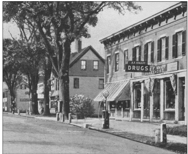
Above: Postcard detail of Knapp's Drug Store in the Brick Block on Main St.
